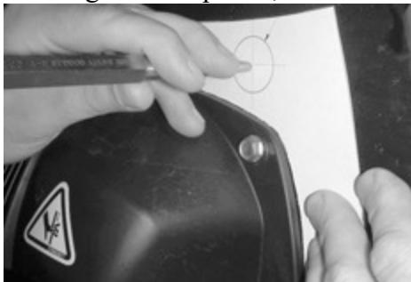
typical -Marking center of hole to drill
